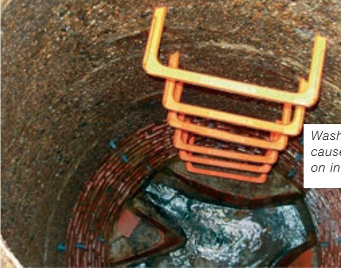
*Washed concrete look caused by acid corrosion in a manhole.*
