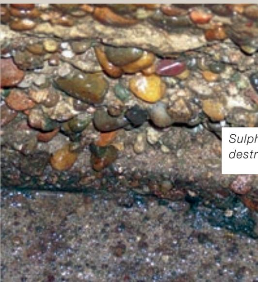
*Sulphuric acid has destroyed the concrete.*
